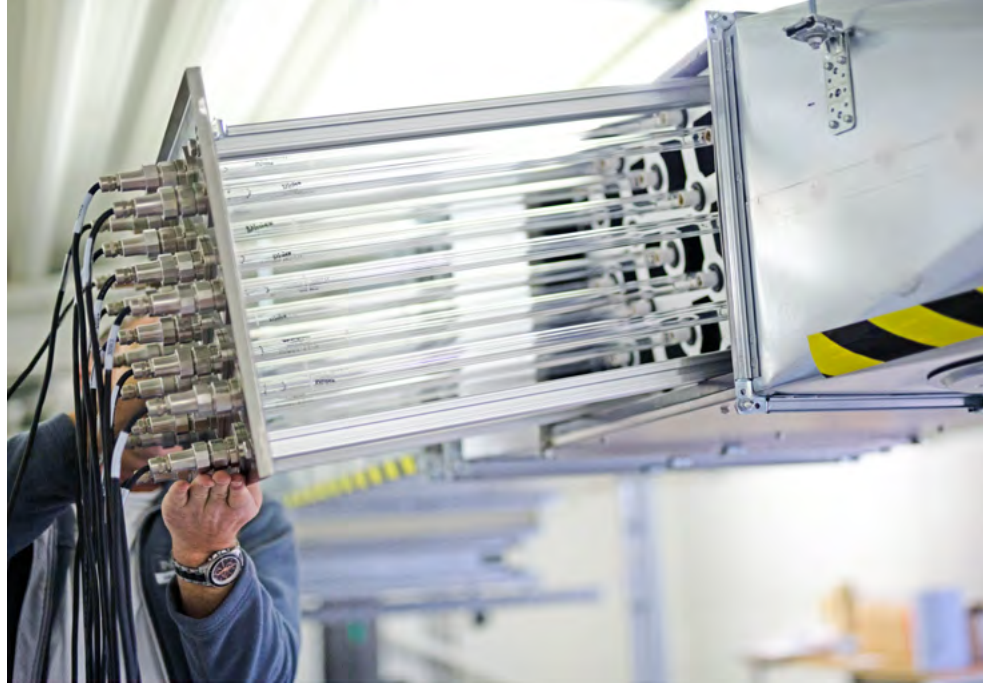
UVC lamps can also be integrated into ventilation systems to improve overall hygiene
