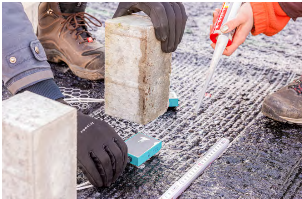
Once the asphalt has hardened, the heavy bricks can be removed
