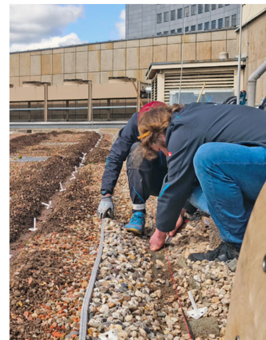
Researchers install fibre-optic cables in and on the substrate of the new Gewandhaus green roof. The cables monitor temperature and moisture, providing early warning signs of drought stress
