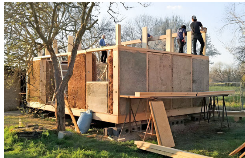
Timber and straw can be used to create load-bearing walls
