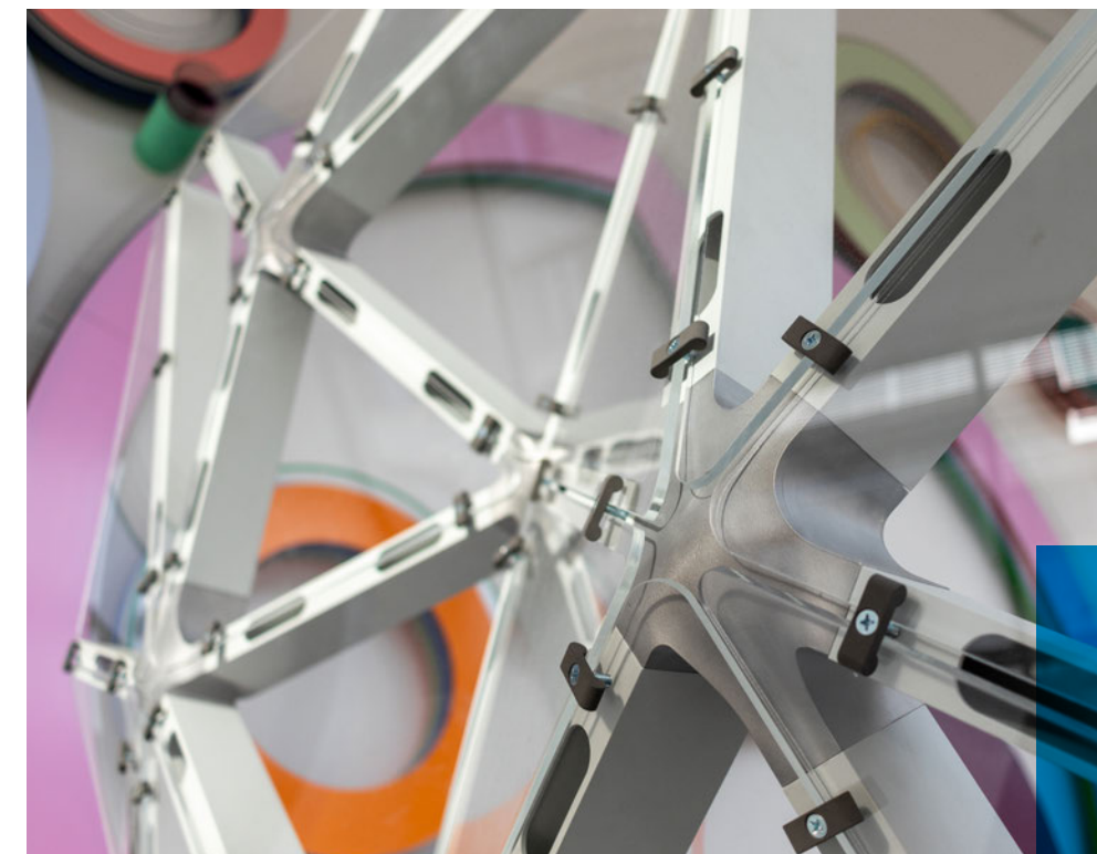
The 3D-printed steel node holds the structural framework
