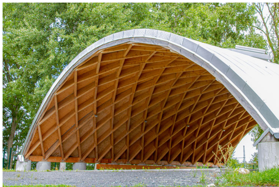
The ribbed structure of the Zollinger roof is not just pleasing on the eye – it also helps to conserve resources
